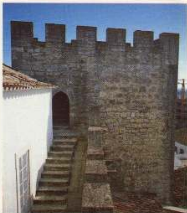
Acceso à sala da torre 1 - Access to the room of the 3rd tower
