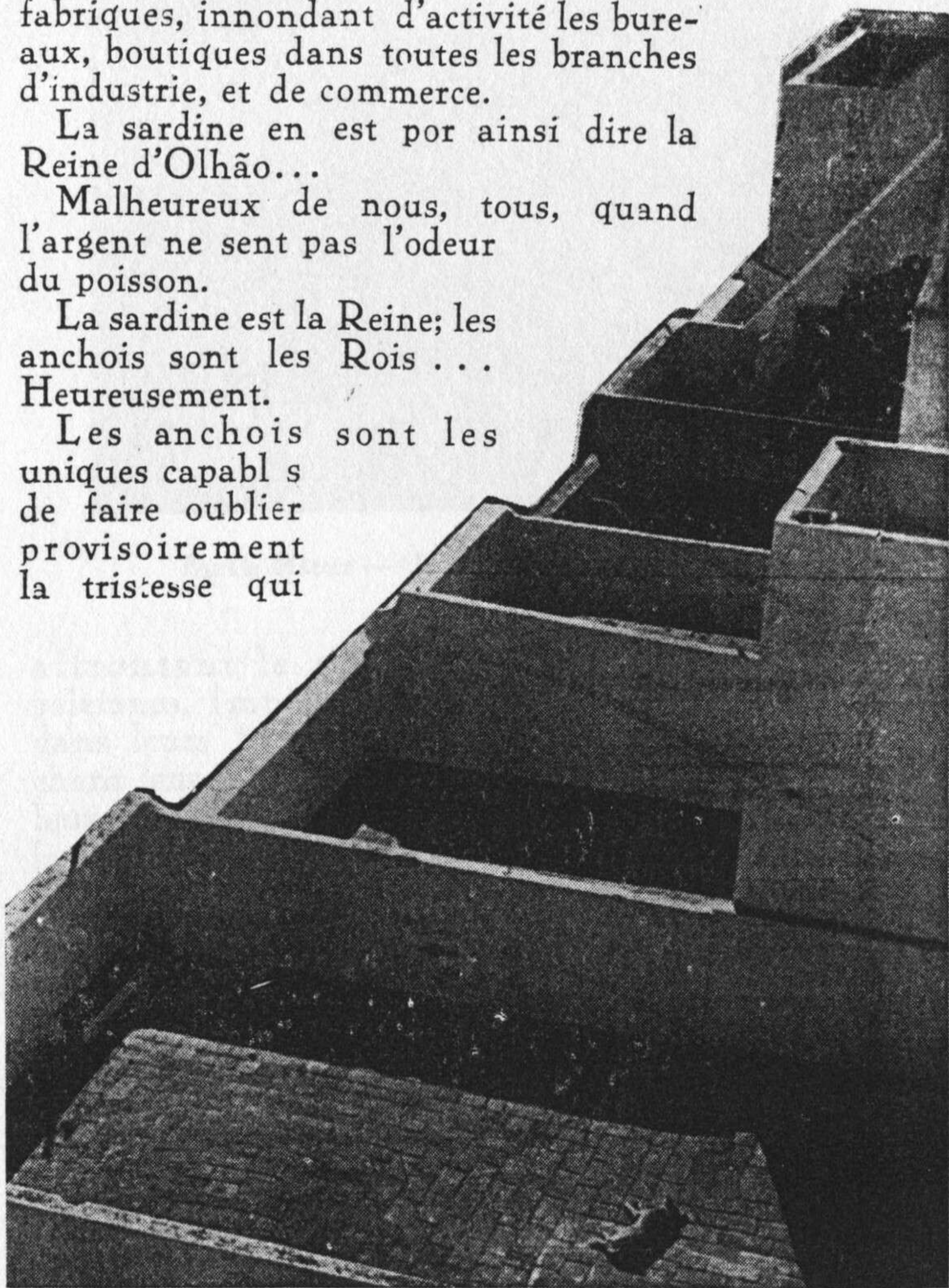
Açoteias — (Terraces of buildings)
